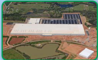
New Cherokee Co., South Carolina distribution center scheduled to begin shipping in June 2016.
