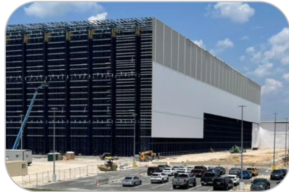
Highly Automated and Engineered
